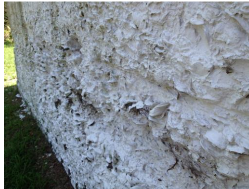
Tabby is made by burning oyster shells to create lime, then mixing it with water, sand, ash and broken oyster shells.
